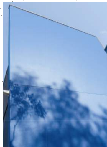
CON01 PRECAST CONCRETE PANELS
