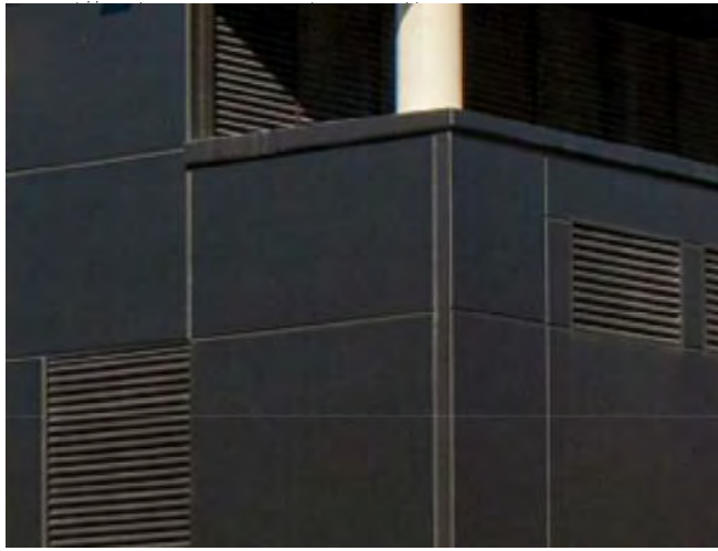
CON02 CONCRETE STRUCTURE GREY
