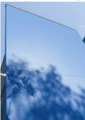
CON01 PRECAST CONCRETE PANELS
